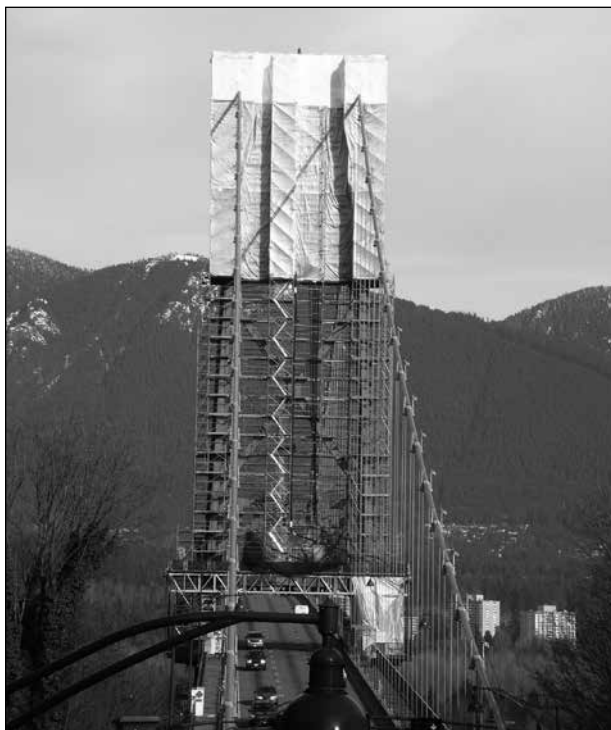
Enclosure containing a lead removal operation on a bridge
