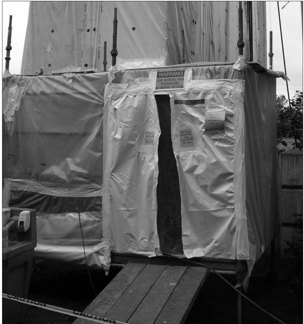
Entrance enclosure for lead removal
