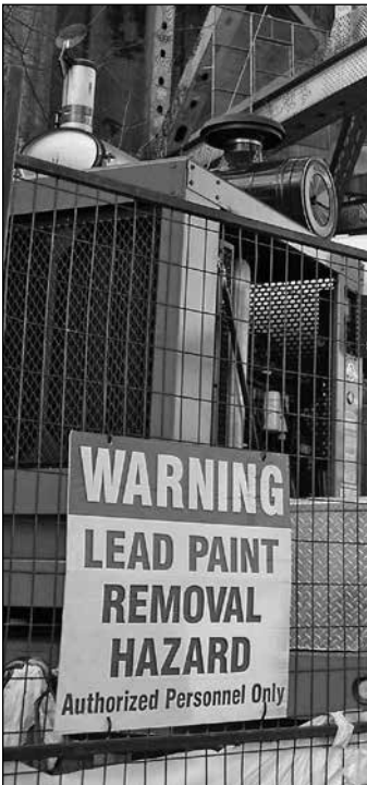
Warning sign on a lead removal site
